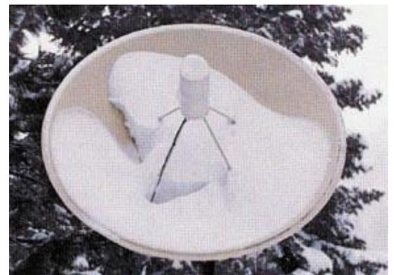
Repeated heavy snowfalls will stretch the panels of mesh and perforated dishes, reducing the accuracy of the reflective surface. Particularly heavy snowfalls will cause the panels to pop out of the channels, and can actually bend the mounts. The added weight of snow puts unnecessary stress on the actuator and motor, and can cause premature failure of either or both. A Satellite Dish Cover will prevent a heavy accumulation of snow and avoid these problems.
